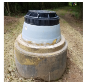
Fiberglass Manhole Insert Installed
