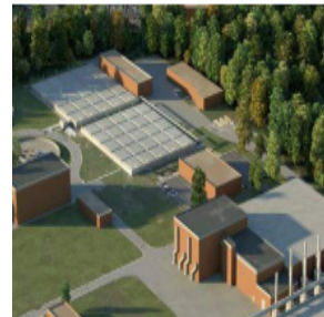
Big Creek WRF Expansion Project Update
