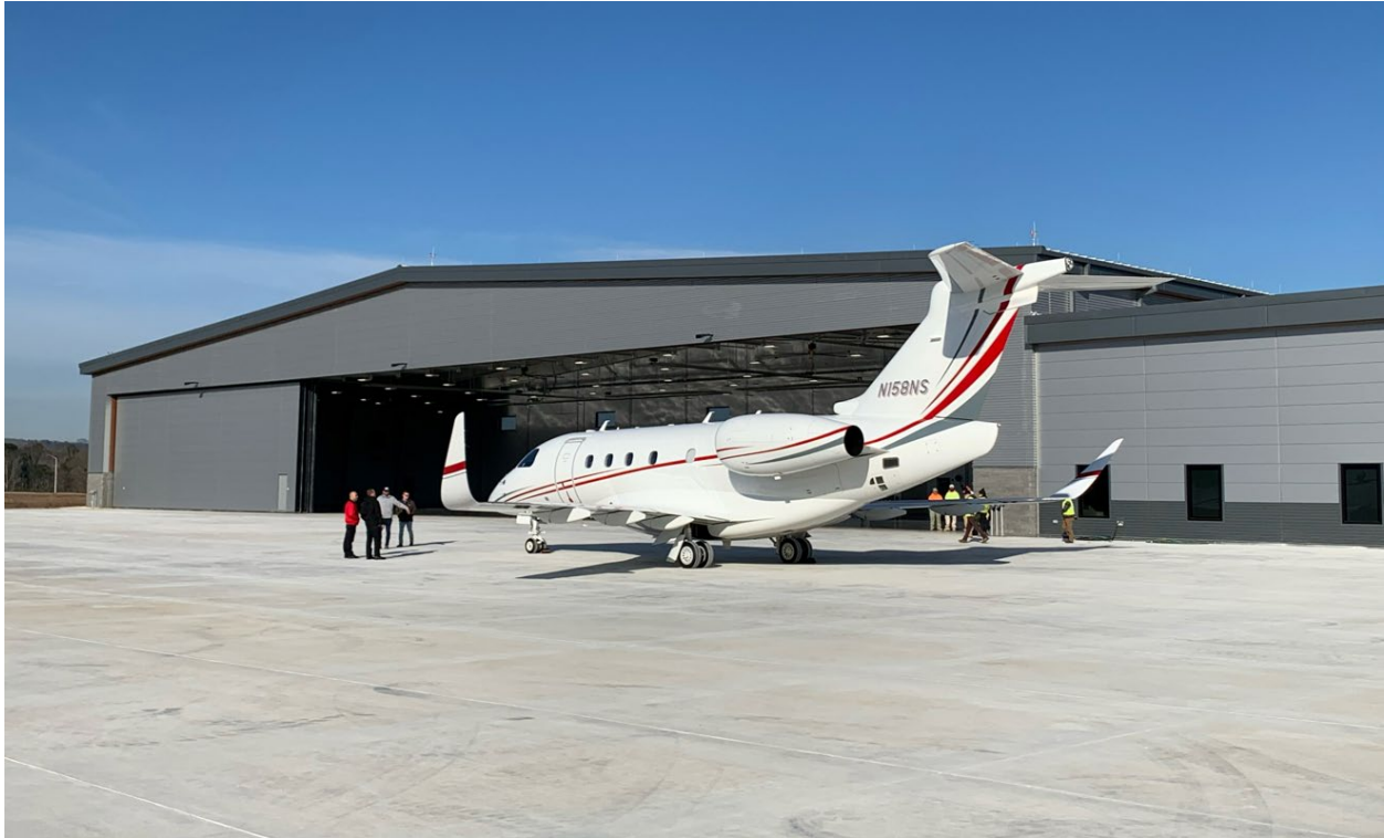
Figure 2-13: Norfolk Southern Corporate Hangar (North Terminal Area)
