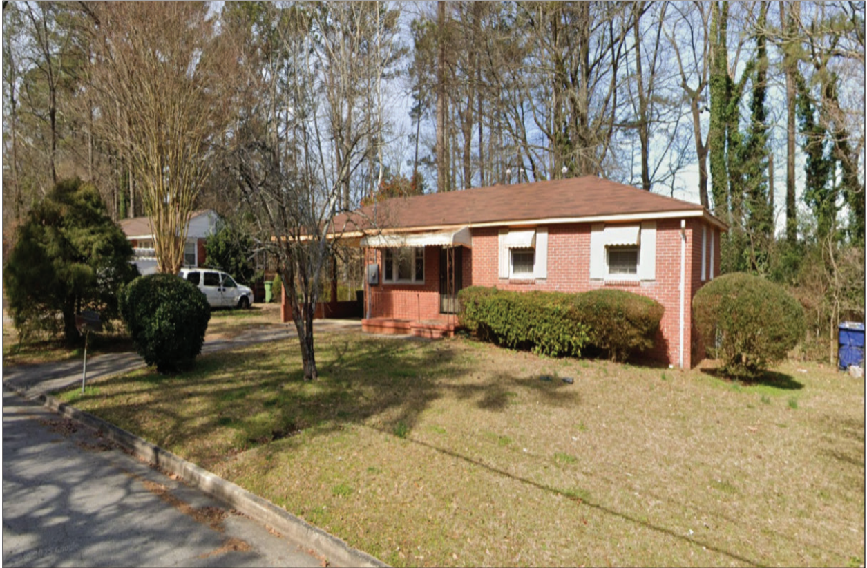
Figure 4.22 Linear Ranch house with hip roof, picture windows, aluminum awnings, and carport; 983 Fairburn Road NW, southeast front elevation.
