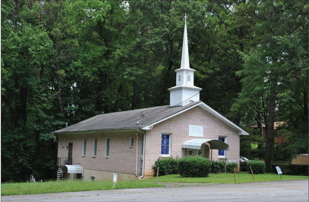
Figure 4.29 C. 1968 Saint Lukes AME Church; Bolfair Drive NW, south front elevation.
