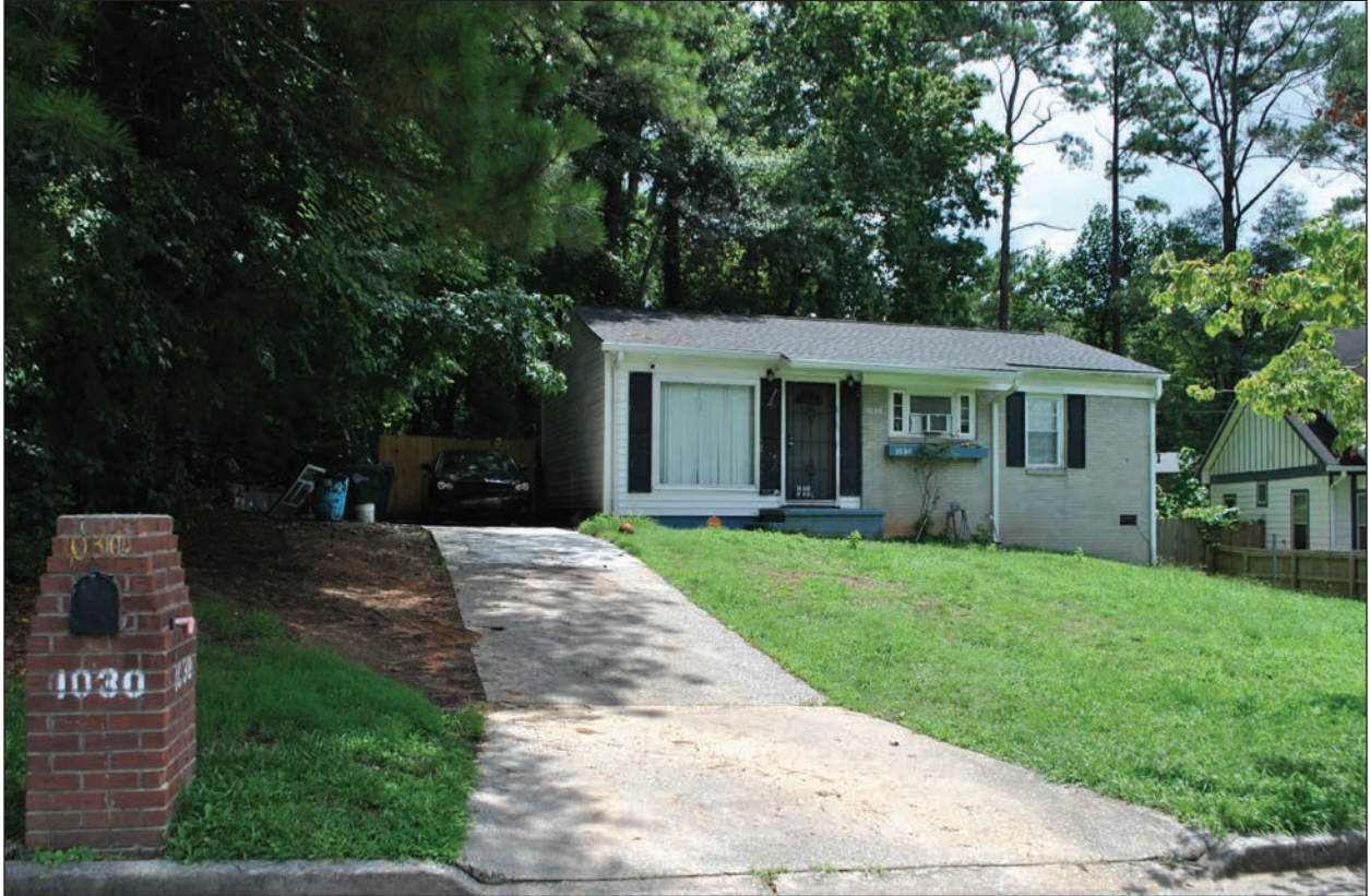
Figure 4.15 Compact Ranch house with picture window; 1030 Fairburn Road NW, southwest front elevation.
