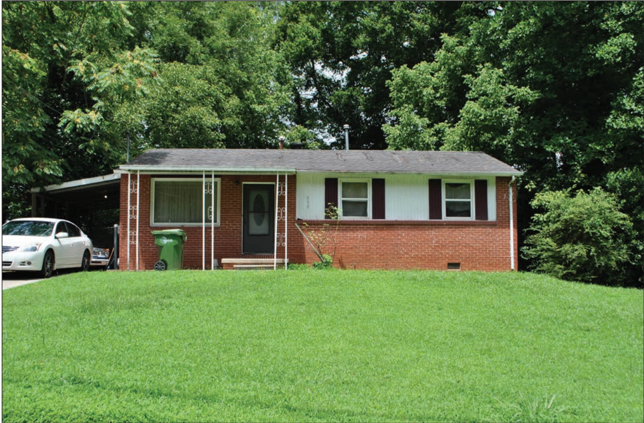
Figure 4.16 Compact Ranch house with picture window, historic aluminum portico, and metal shed-roof carport addition; 899 Fairburn Road NW, northwest front elevation.
