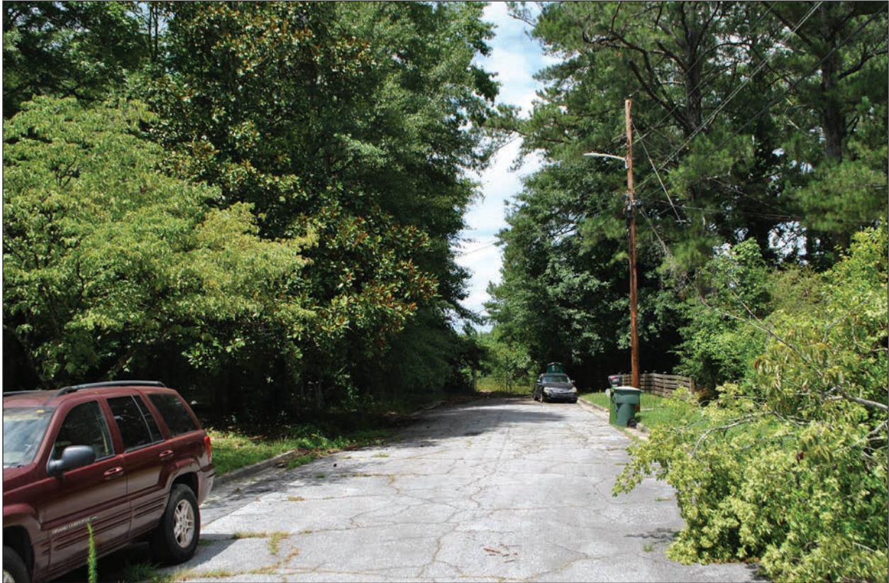
Photograph 5. 2024 photograph of Neptune Place NW, looking northwest toward the proposed grading area/ borrow pit.
