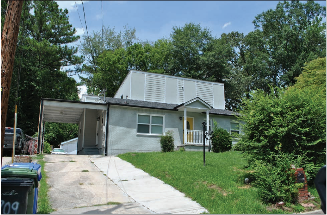
Figure 4.26 Compact Ranch house with c. 2020 second story addition; 3709 Clovis Court NW, south front elevation.
