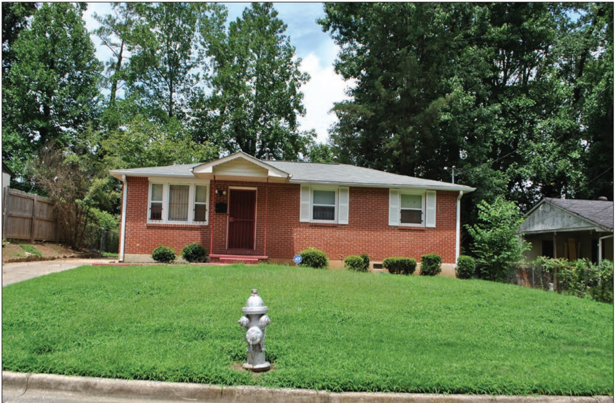
Figure 4.18 Compact Ranch house with hip roof and picture window; 929 Fairburn Road NW, south front elevation.
