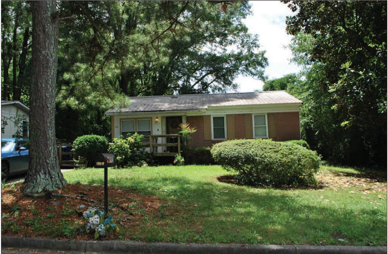
Figure 4.14 Compact Ranch house with no carport and V-crimp metal roof; 1092 Fairburn Road NW, northeast front elevation.
