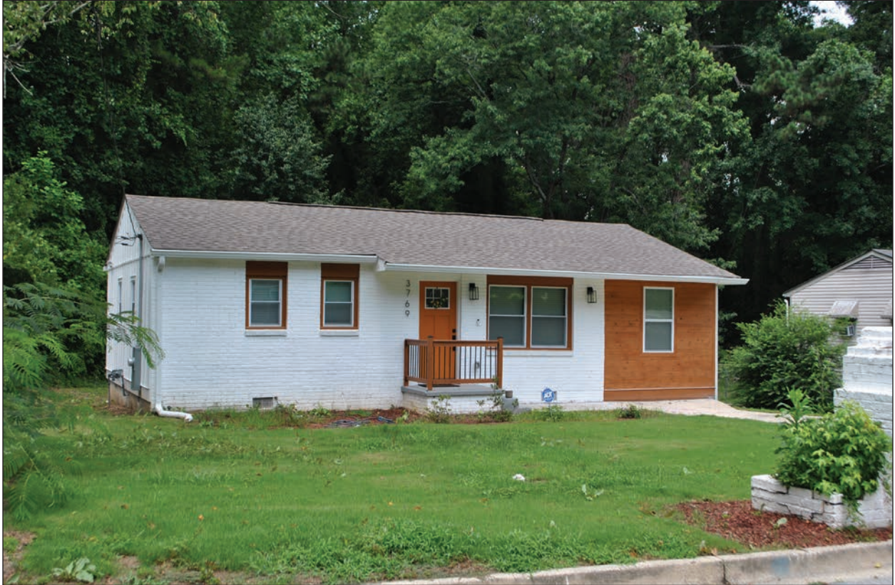
Figure 4.17 Compact Ranch house with replacement windows and enclosed carport; 3739 Adkins Road NW, south front elevation.
