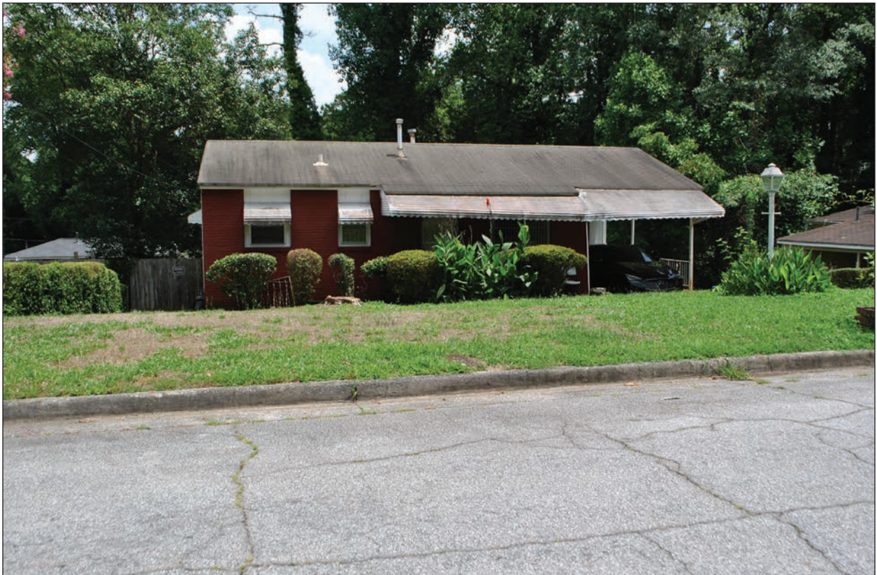
Figure 4.19 Linear Ranch house with integral carport and aluminum awnings; 763 Amber Place NW, west front elevation.
