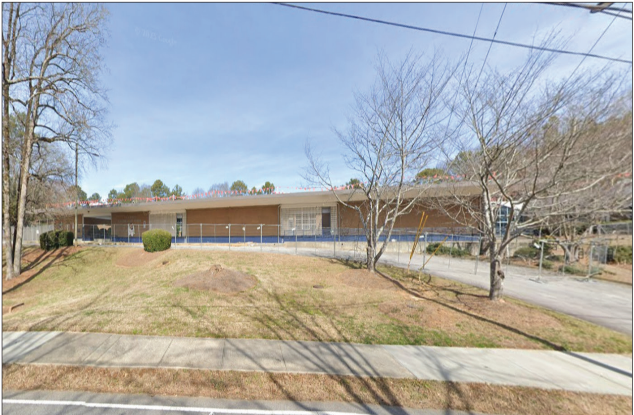
Figure 4.27 C. 1968 former G.A. Hill Elementary School building; 749 Bolton Road NW, south front elevation.
