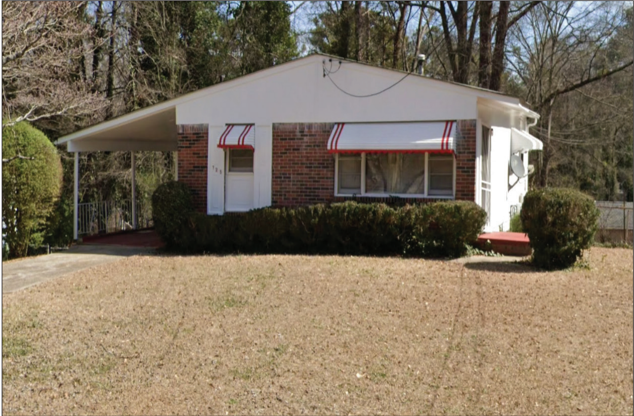
Figure 4.24 Contemporary Ranch house with picture window and integral carport; 725 Amber Place NW, west front elevation.
