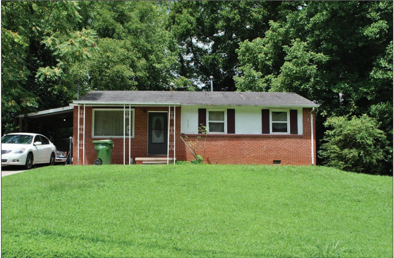
Figure 4.16 Compact Ranch house with picture window, historic aluminum portico, and metal shed-roof carport addition; 899 Fairburn Road NW, northwest front elevation.
